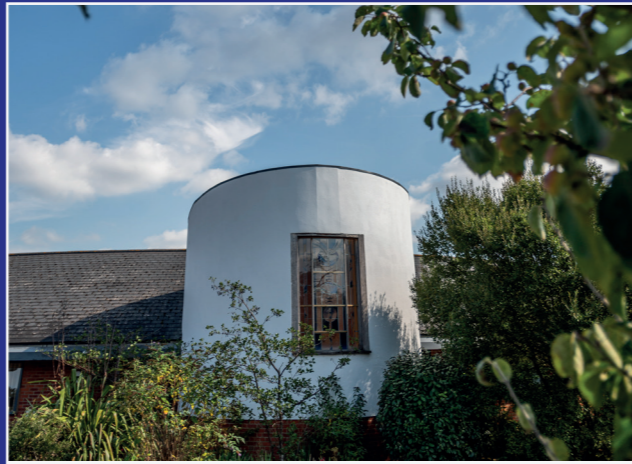
The chapel exterior
